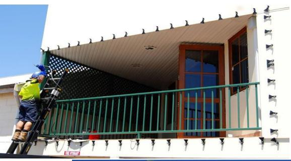
This balcony has anchors in the concrete and welded onto the metal beam.
