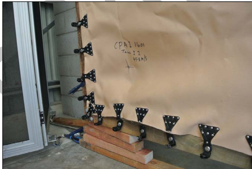
Figure 8: General view of impacted area
