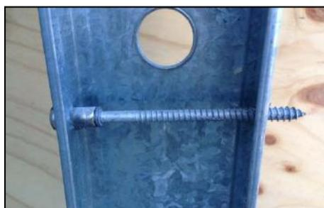
**Figure 12:** Photograph of a threaded screw anchor installed into the C-channel of the steel support frame for Trial I6
