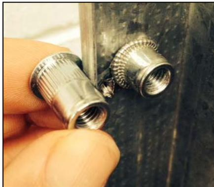
**Figure 11:** Photograph of two threaded hollow rivets used in the steel support frame, one prior to installation and the other installed into the steel support
