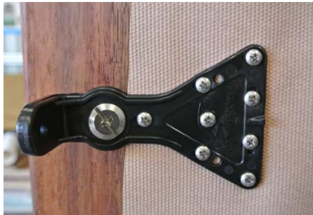
Figure 3: Typical assembled clip installed to Astrogard screen fabric
